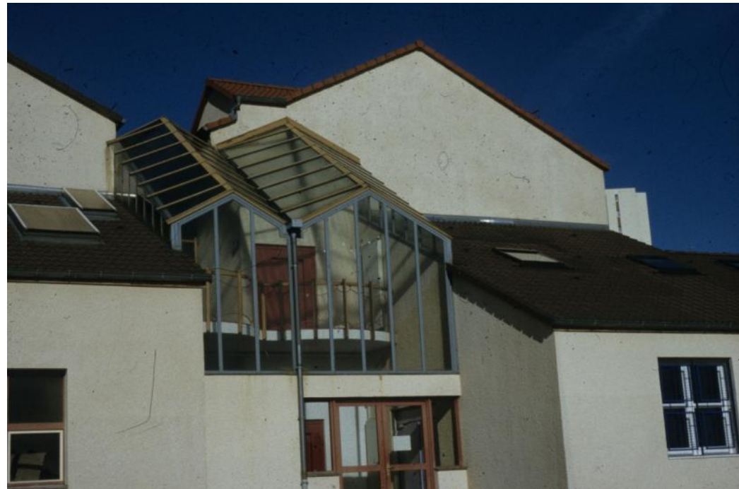
Belfort-Bethoncourt (F). School
