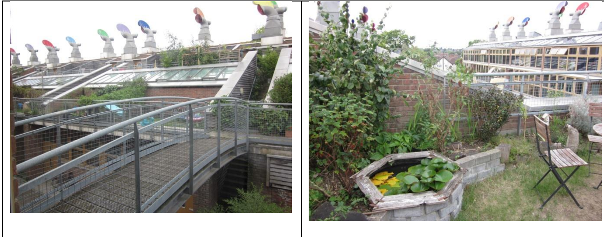
Figure 21 : London (UK): Density (and compactness) of dwellings in Beddington zero fossil energy development (BedZED) is higher than in traditional garden-cities. The developer moved away from the traditional single detached houses towards more density.
