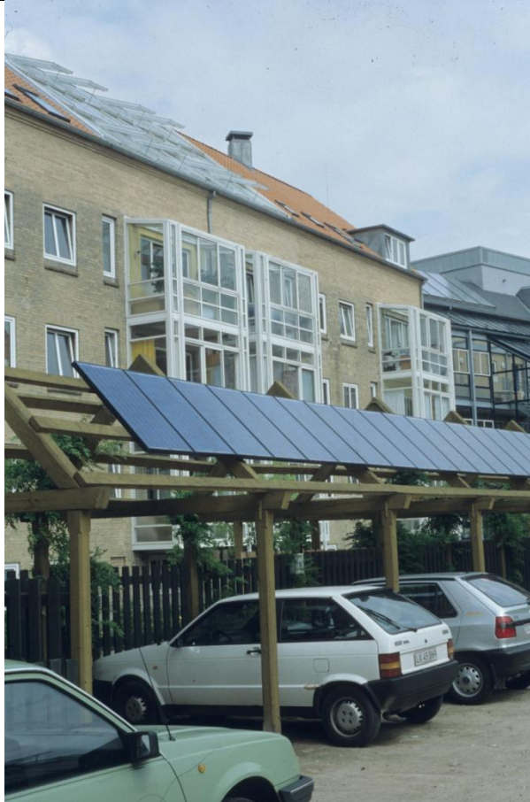
Kolding (Denmark). Common car ports with a photovoltaic energy plant on the roof, built in the semi-public parts of this urban building block. Picture by Erik Rombaut
