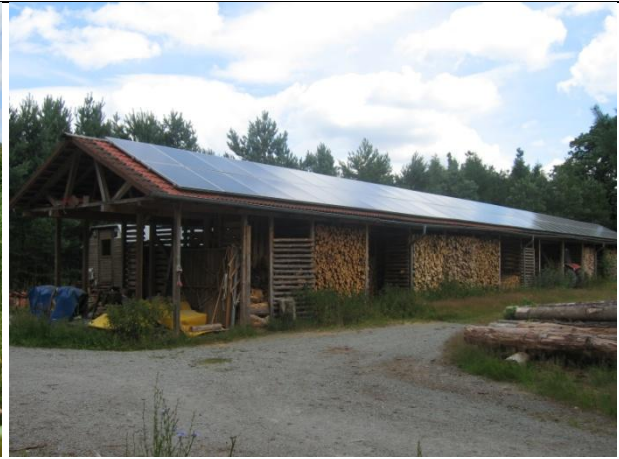
Poppau (Germany): Common wood stock and a collective photovoltaic plant in the ecovillage Sieben Linden . Picture by Erik Rombaut
