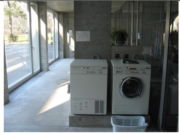
Zürich (Switzerland). On the ground Floor a lot of common functions are designed, for example this common laundry, stimulating social cohesion in this Werdwies project. Picture by Erik Rombaut
