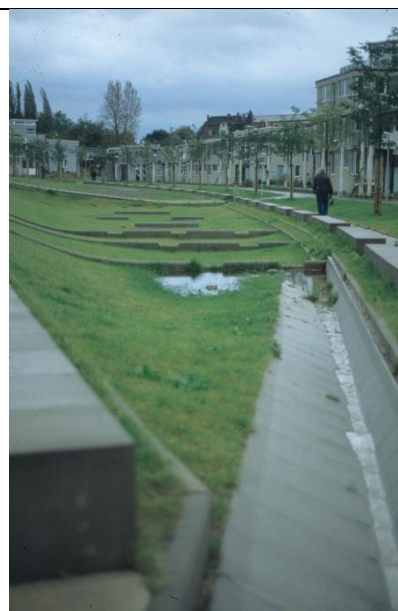
Gelsenkirchen (Germany). Infiltration zone in the ecoquarter Koppersbusch . Picture Erik Rombaut
