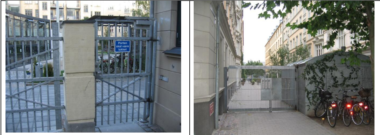
Copenhagen (Denmark). Fences make the inner green areas inaccessible for the public in the Hedebygade project. Picture Erik Rombaut.
