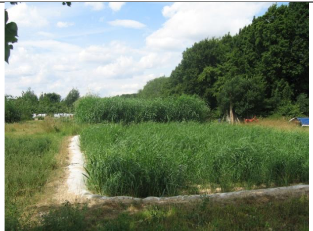
Poppau (Germany): By using compost toilets the surface needed for the plant purification system can be minimised (only grey water) in the ecovillage Sieben Linden . Picture by Erik Rombaut
