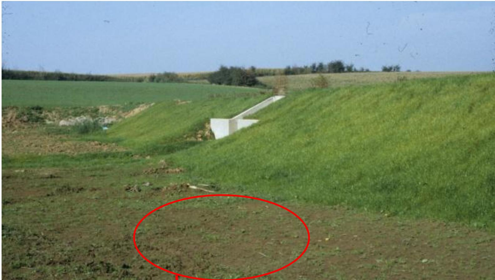
Hoegaarden (B). Building a dam across the stream, with a narrow passage structure is needed to create a temporary storage basin.
