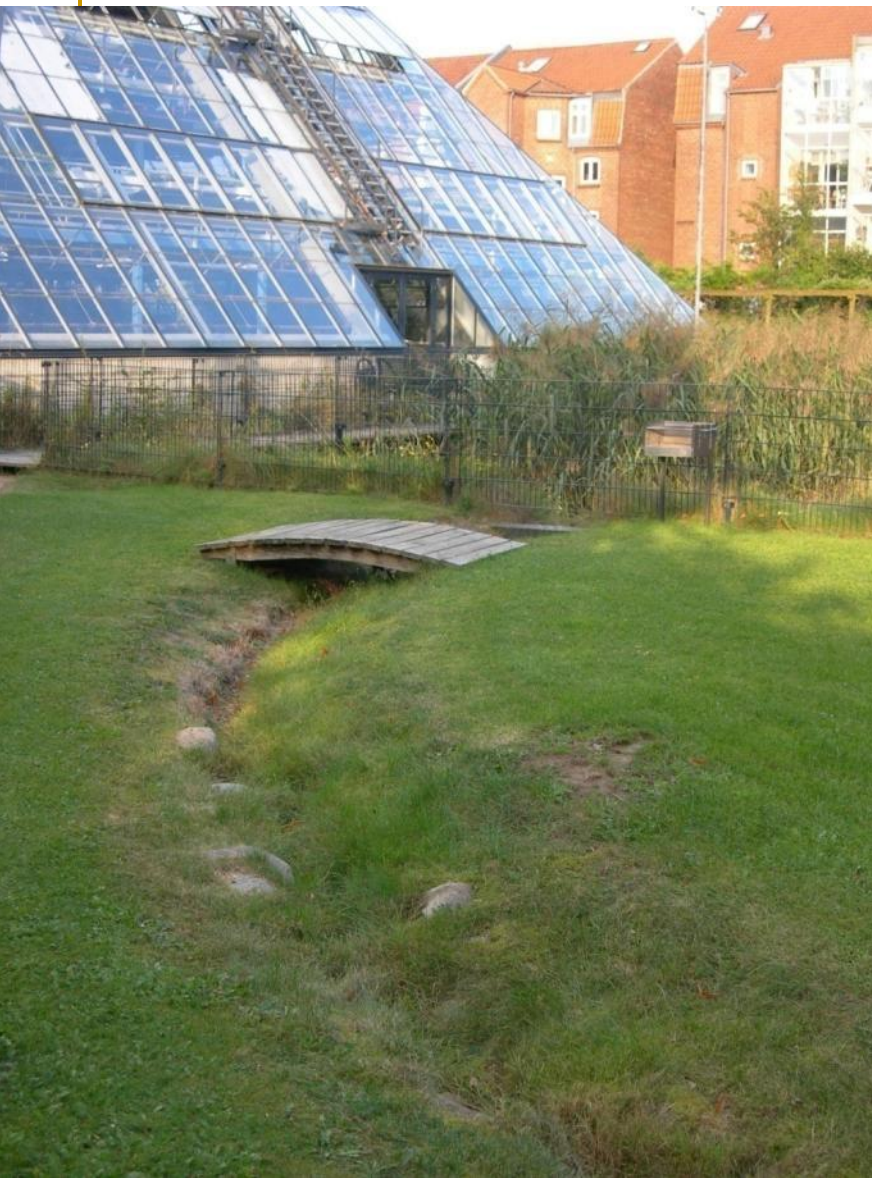
Wadi for infiltration of white water
