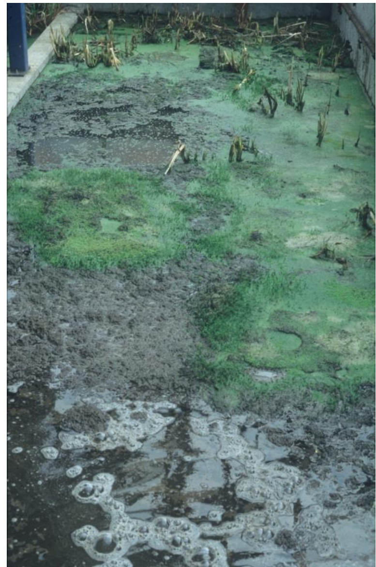
Black and grey water are purified in a plant purification system.
