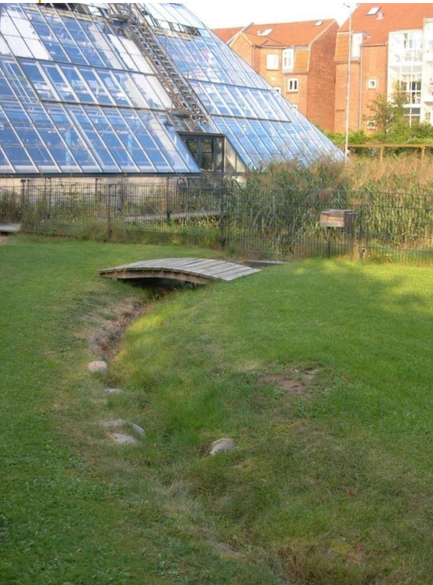
Wadi for infiltration of white water
