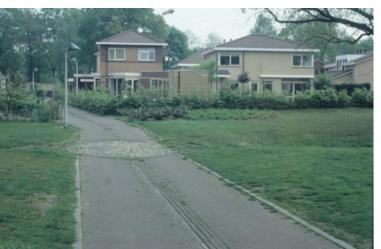
The 'slokop' is connected with the sewage system and prevents flooding.
