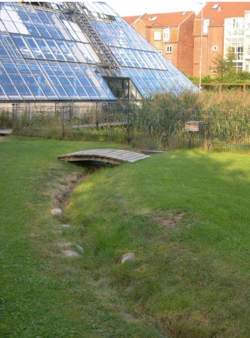
Wadi for infiltration of white water
