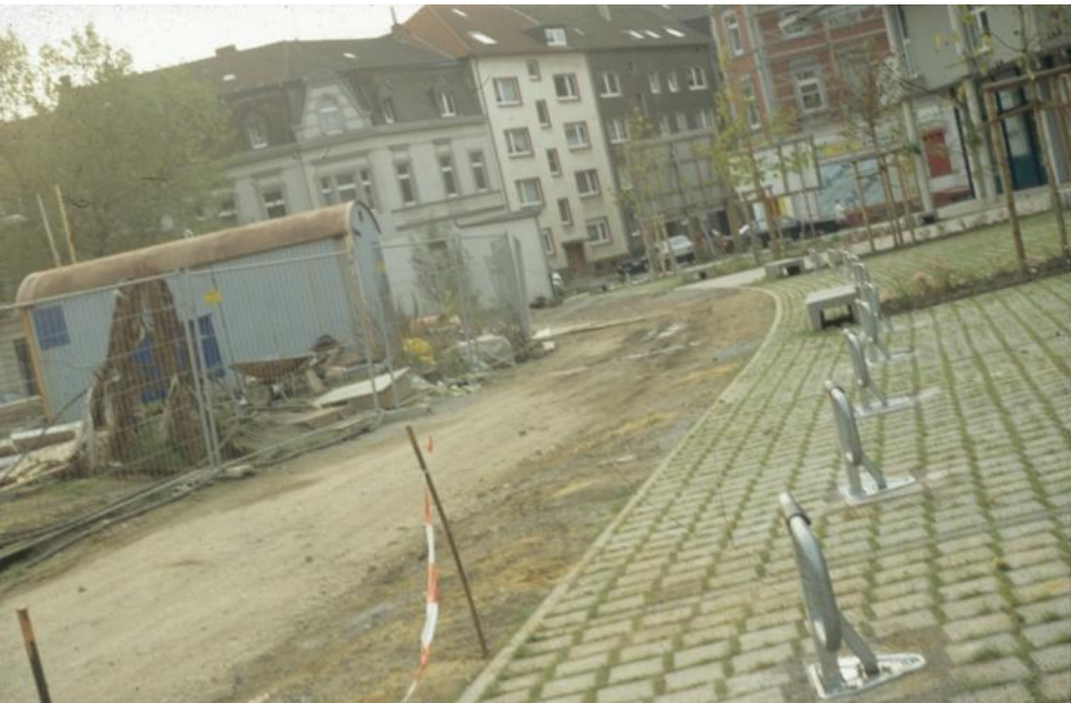
Permeable parking area
